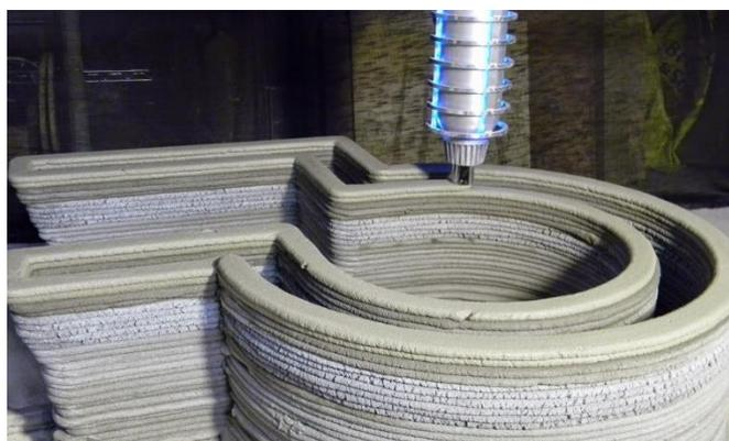
Figura 5 - Concrete Printing. Fonte: LIM et al. (2012)
