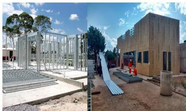
Figura 10 – Alvenaria vs Light Steel Frame
